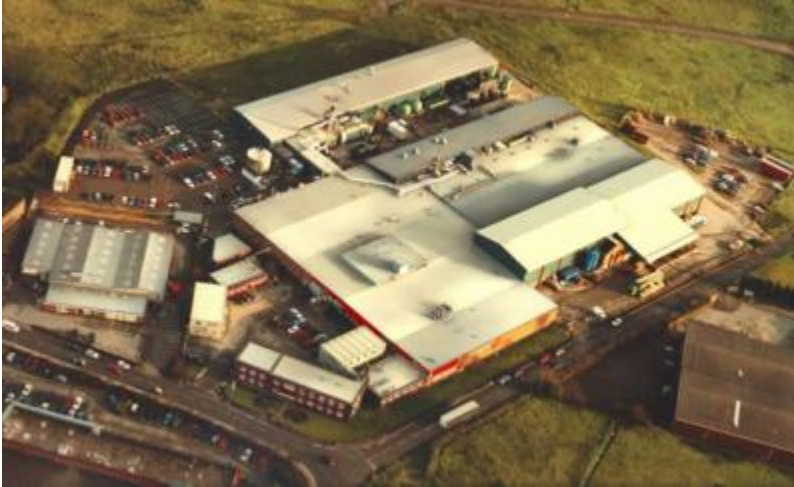
Kodak GCG plant in Leeds
